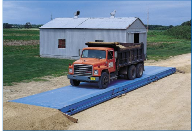
ABOVE: Portable truck scale installation with temporary gravel ramps.
